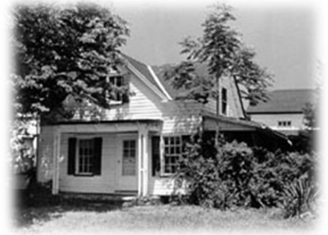
The Grimes House in Boonton
