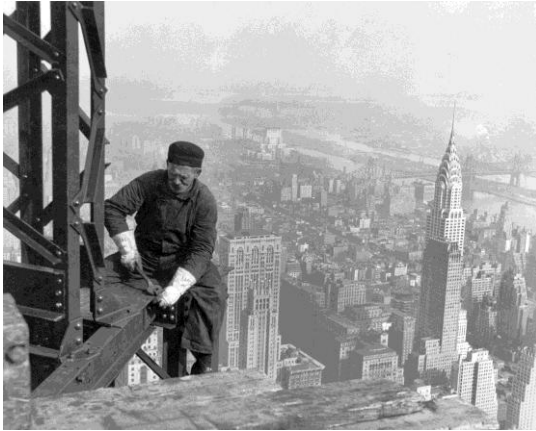
Construction on the Empire State Building
