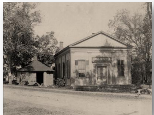
Early Borough Office and Jail and formerly the Presbyterian Sessions House
